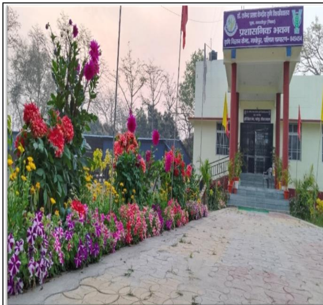
KVK administrative building
